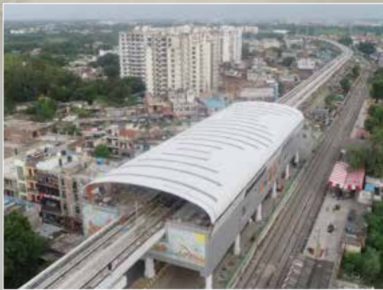
Kanpur Metro wins a double CIDC Viswakarma Awards 2022, Excellence in Infrastructure & Civil Works at Rail Analysis India Summit 2022
